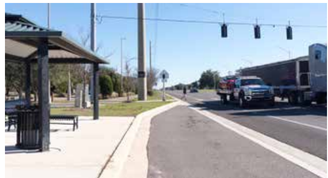
The two photos above are from the same roadway and illustrate an example of a high-volume roadway that balances the needs of freight traffic, transit, and pedestrians and bicyclists of varying abilities. The corridor includes a shared use path, bicycle lanes, bus pull-outs, bus shelters with benches, and other amenities. Location: US 98, Polk County, FL Source: KAI
